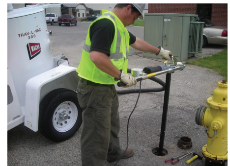
Highly portable handheld design allows operation of valves from 6-60in
